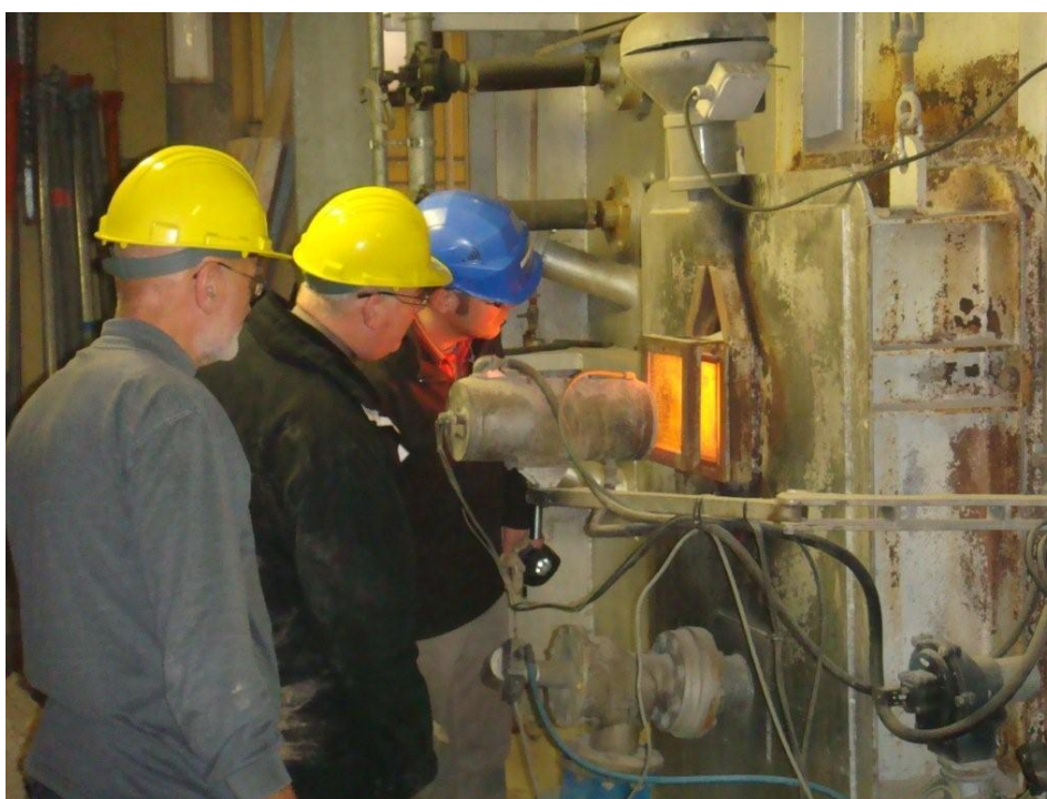
From the IVM WtE Plant in Eeklo, Belgium
