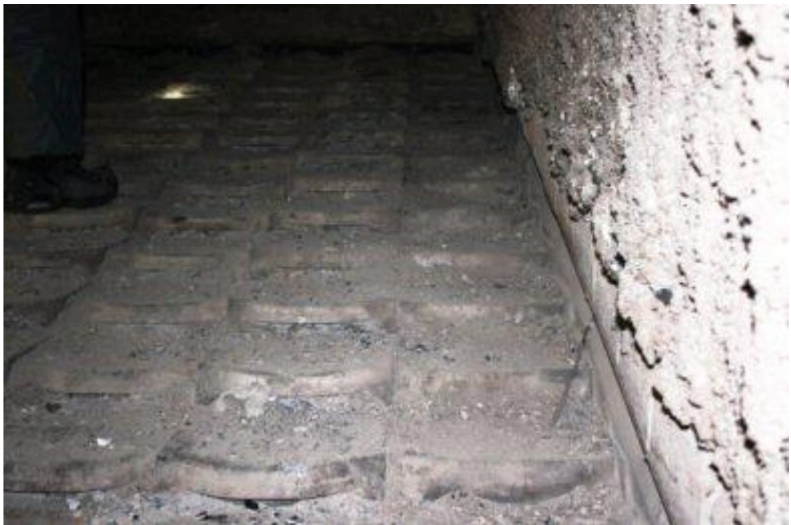
Photo 14 inspection after 4 month's operation shows a tight carpet surface
