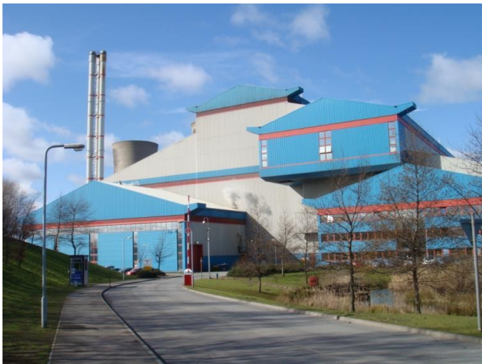
Photo 19 SITA Tees Valley (UK) Installation on 2 lines, May & September 2011
