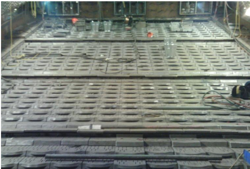
Photo 13 Tees Valley (UK), almost finished grates 2.5.2011
