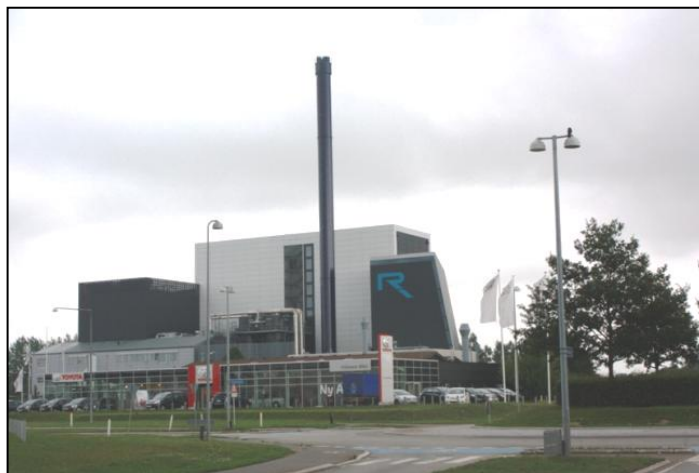
Photo 3 The I/S REFA plant in the south of Denmark with 3 combustion lines was one of the first installations in Denmark with Type DUB 3 grate
