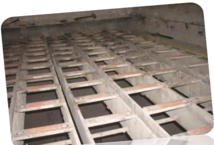
Photo 6 details from an installation in France
