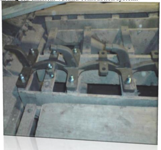
Photo 5, The new Type DUB 3 grate carpet installed inside an existing old classical Vølund combustion system.
