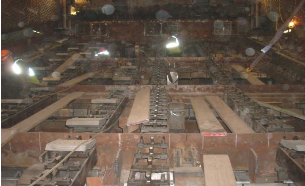
Photo 12 Tees Valley (UK) during erecting
