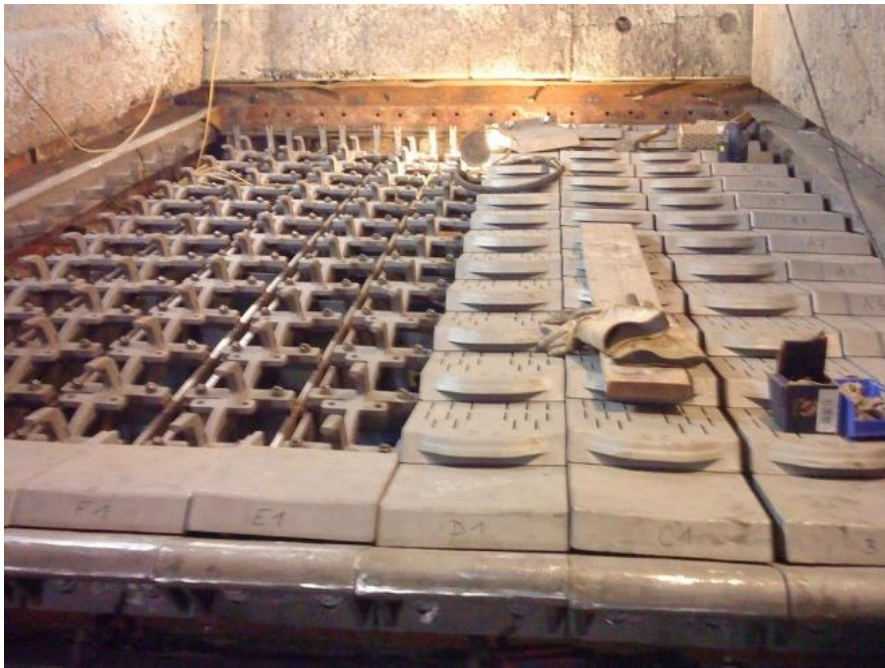
Photo 2 Details from an early grate carpet installation in Denmark
