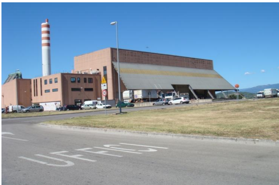
Photo 20 AISA, Arezzo (IT) DUB 3 Installation on 1 line, September 2013-2017
