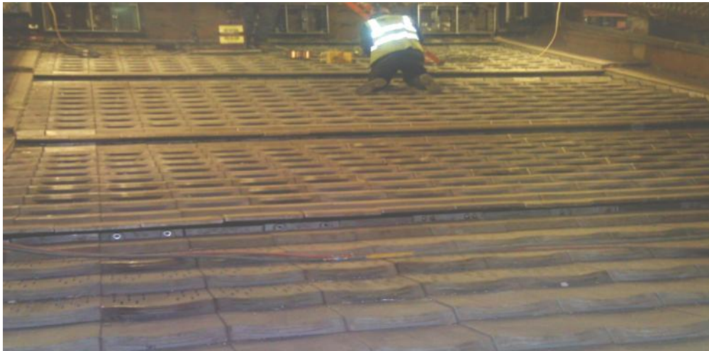
Photo 1 from the installation of DUB 3 grate in Tees Valley, UK, 2011
