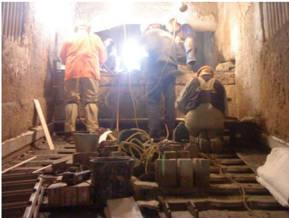
Photo 18 installation at DONG Energy Horsens kraftvarmeværk
